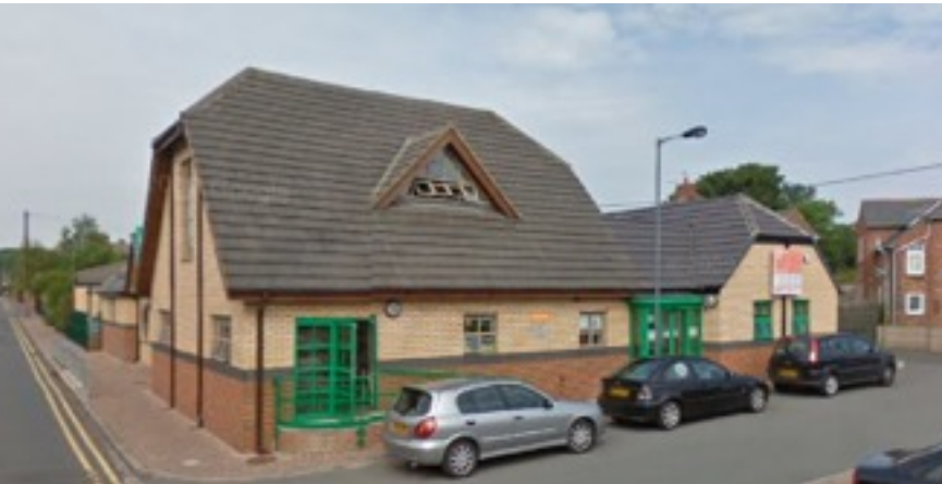
View from the outside of this much extended nursery
